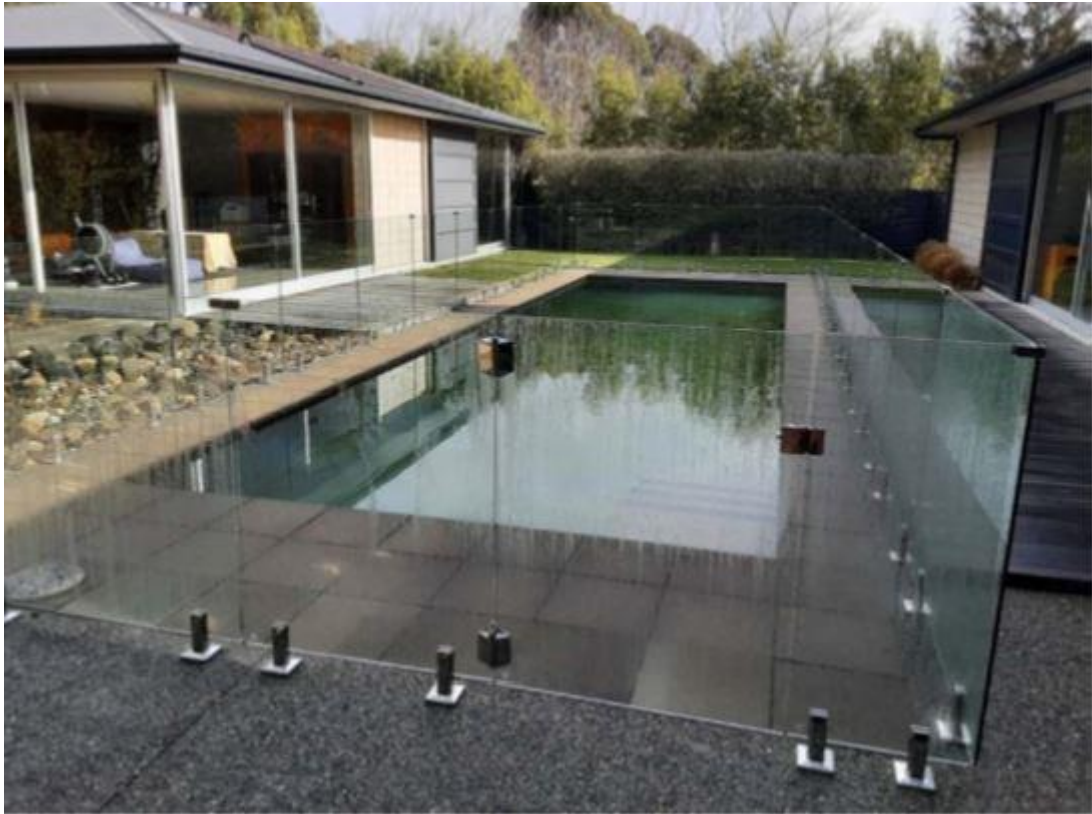
Photograph 2: Pool with compliant barrier
